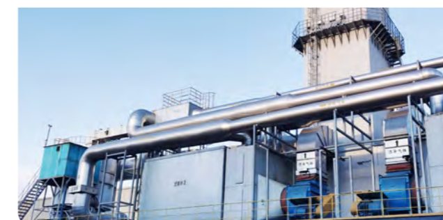
RTO waste heat facility modification
