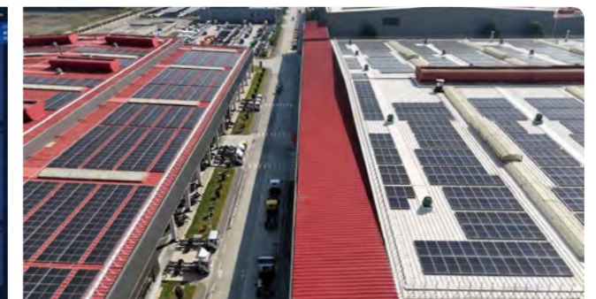
Distributed photovoltaic project development
