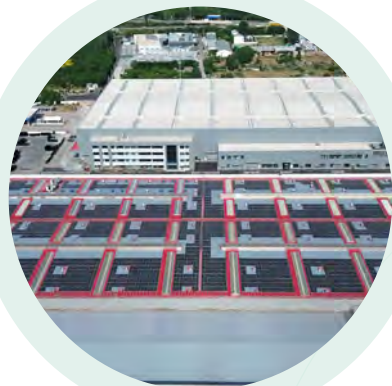
▲ Rooftop photovoltaic installation
